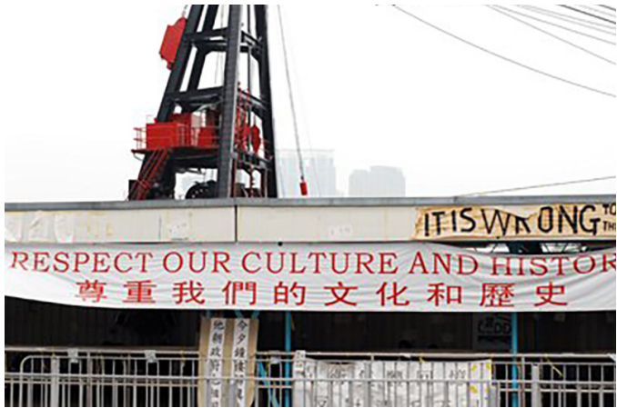
Figure 3: The Central Star Ferry Pier shortly before demolition. 28 (Copyright: Thai World View.) x
